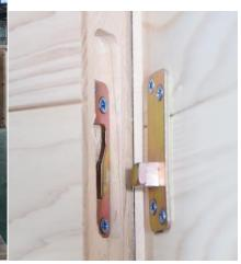
4. Attach the front wall by sliding it onto the wall slide brackets.
