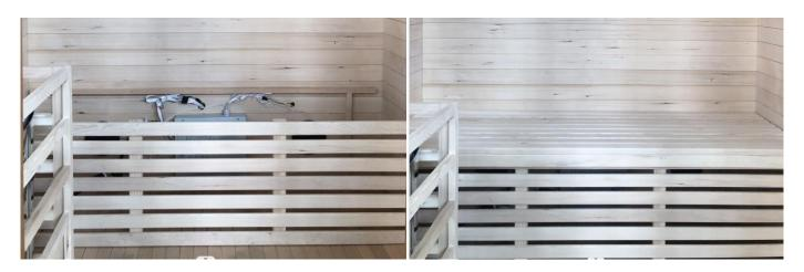
8. Screw the back rest into the back wall and attach the accessories as shown.
